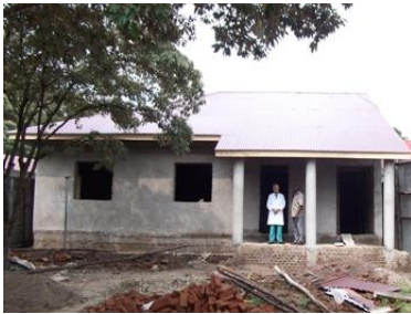
Theatre extension under construction – Jun 2011
